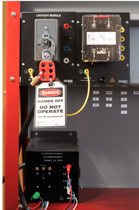
Figure D-4. Installation of padlocks and hasps.
