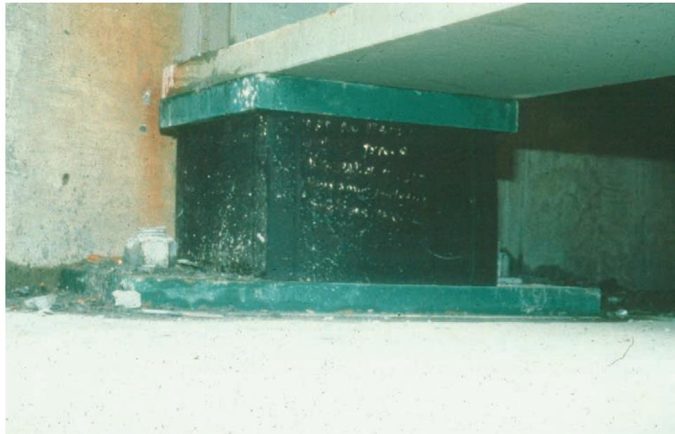
Figure 9.1.16 Lead Core Isolation Bearing
