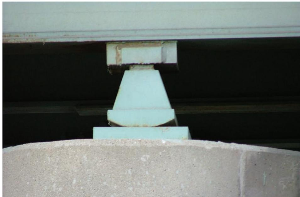
**Figure 9.1.9** Rocker Bearing
