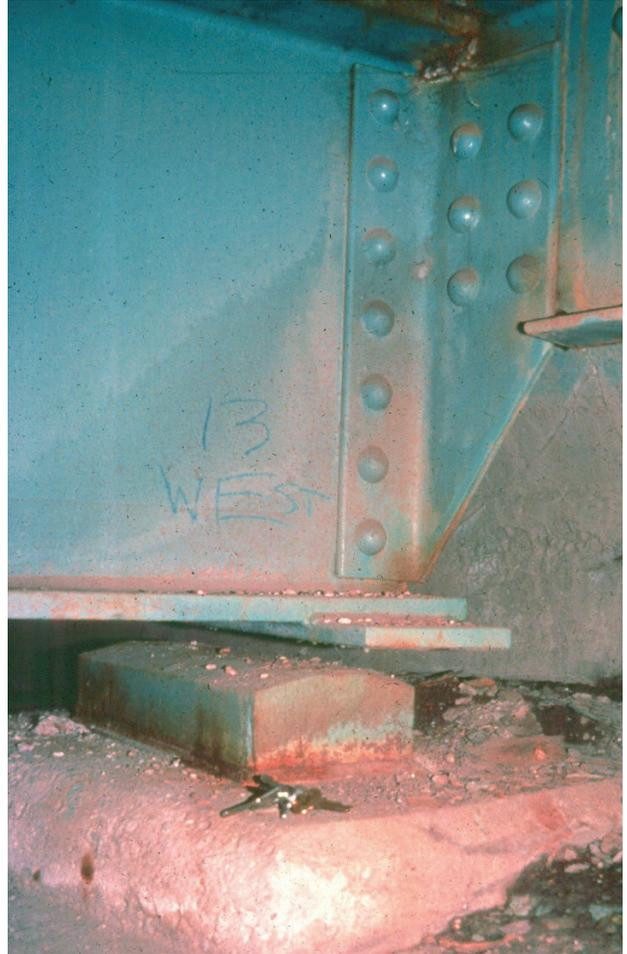
**Figure 9.1.26** Uplift at Bridge Bearing
