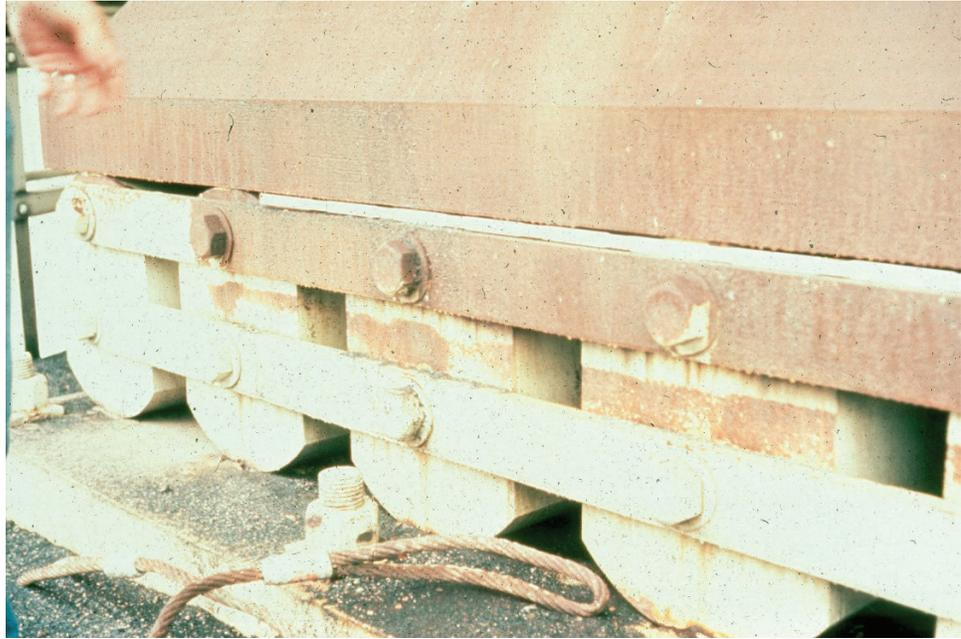
**Figure 9.1.11** Segmental Rocker Nest Bearing
