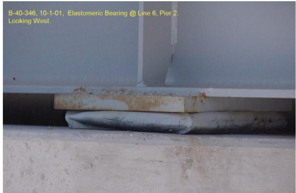
**Figure 9.1.35** Neoprene Bearing Pad Excessive Bulging
