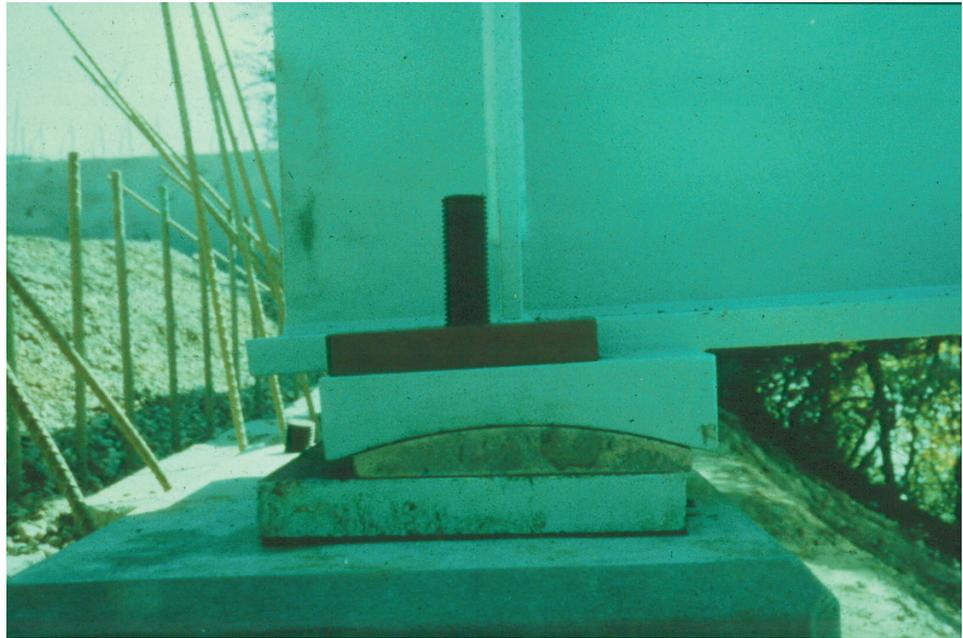
**Figure 9.1.5** Bronze Sliding Plate Bearing
