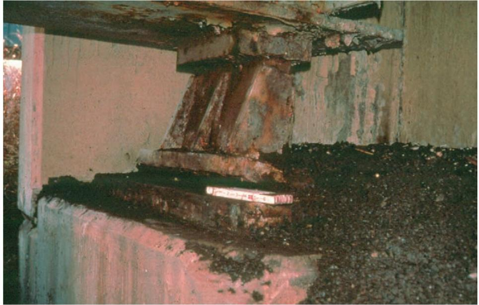
**Figure 9.1.22** Heavy Corrosion and Excessive Movement on Steel Rocker Bearing
