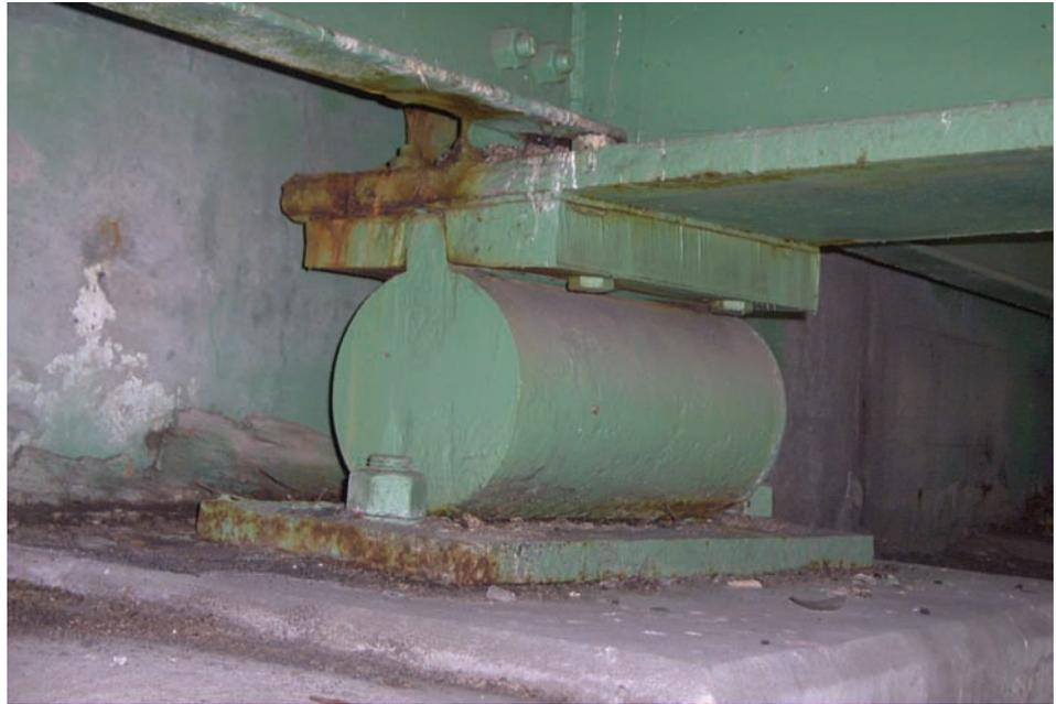
**Figure 9.1.7** Single Roller Bearing
