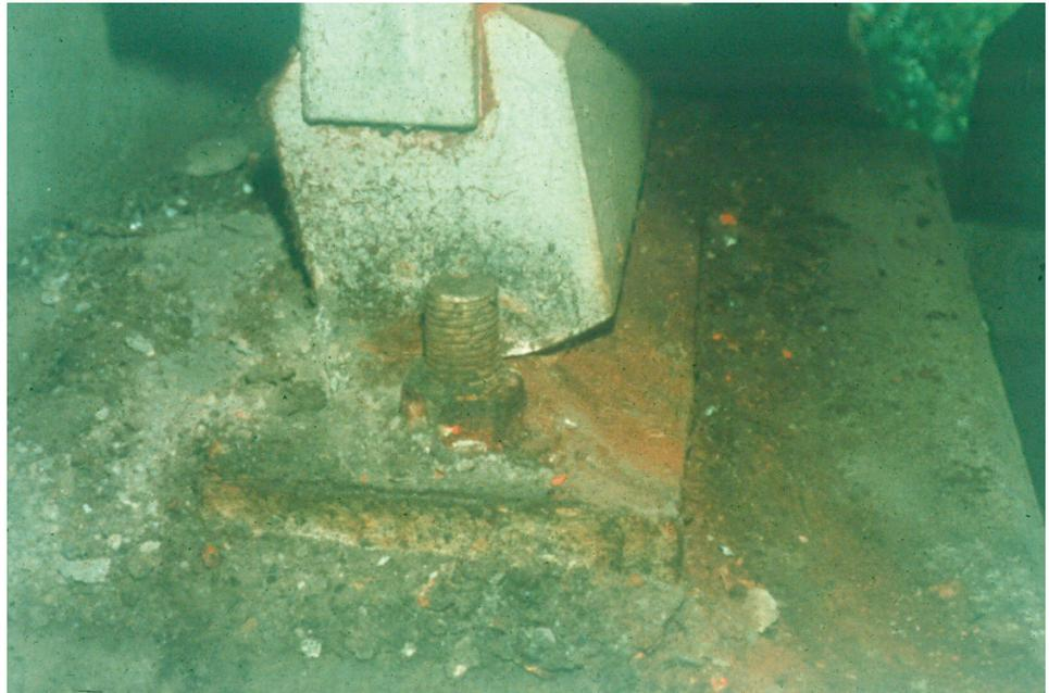
**Figure 9.1.10** Segmental Rocker Bearing
