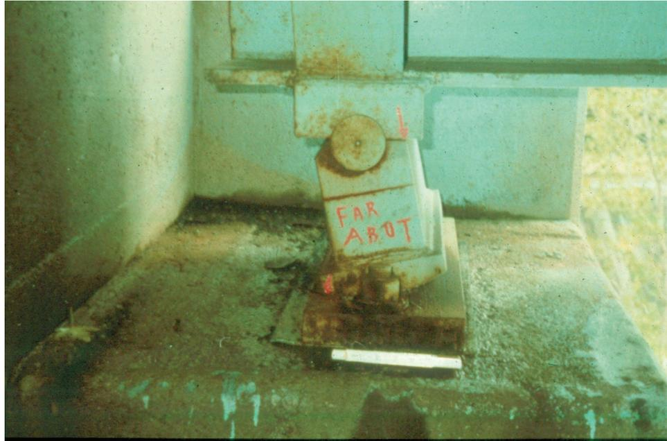
**Figure 9.1.38** Broken Pintle on a Bearing
